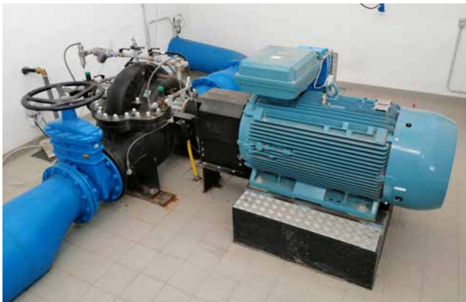
NR. 1 SKDZ-4P 250-560 315kW HIGH EFFICIENCY VERSION WITH PUMP EFFICIENCY > 80% AND ABB IE4 SYNCHRONOUS MOTOR
